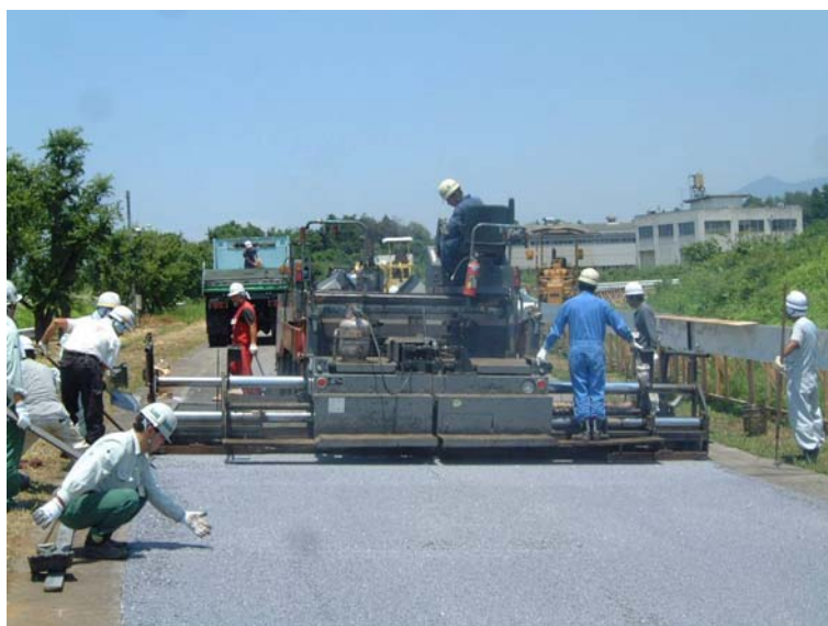
FIGURE 8 View of applying test pavement
