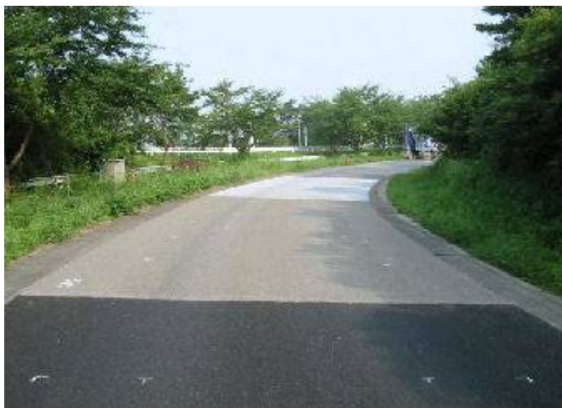
FIGURE 10 View of the completed test pavement
