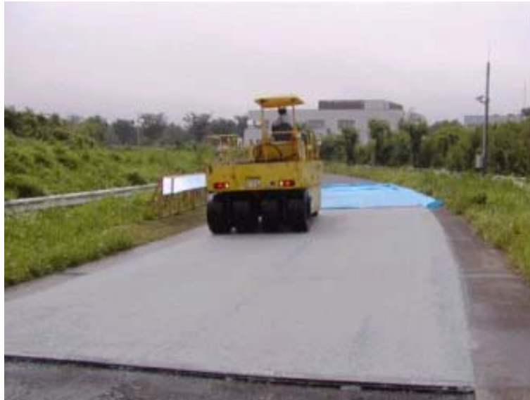
FIGURE 9 View of conducting rolling compaction
